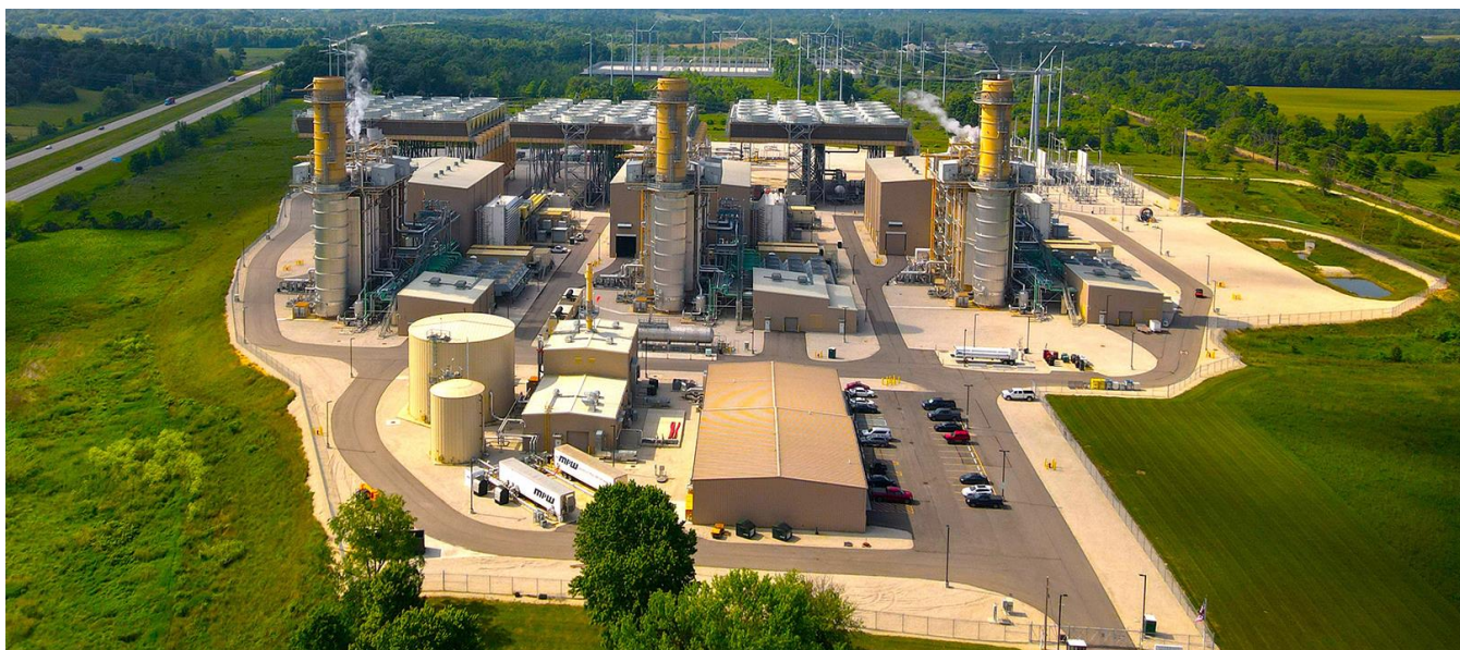
The Guernsey Power Station, image courtesy of Talen Energy
